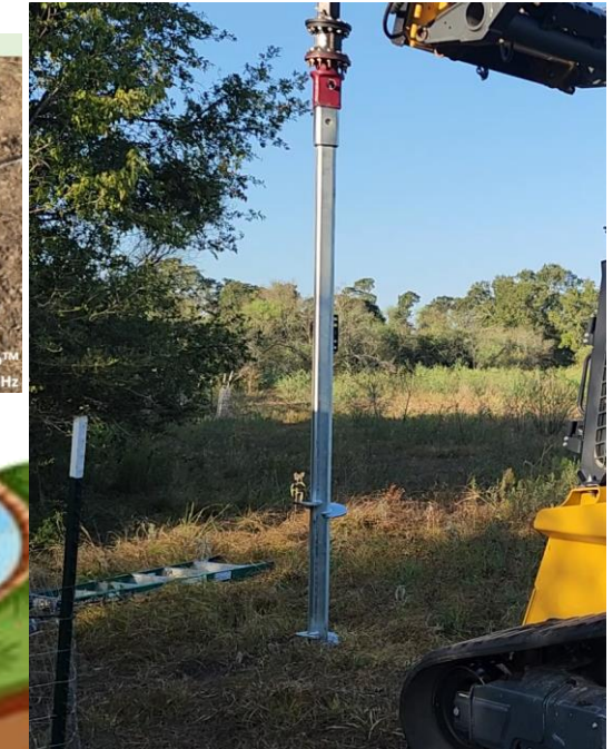
Helical Anchor Installation at Test Site
