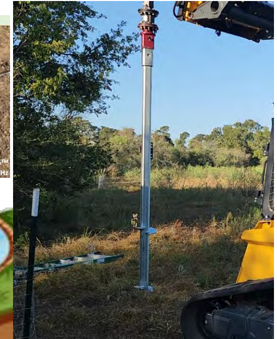
Helical Anchor Installation at Test Site
